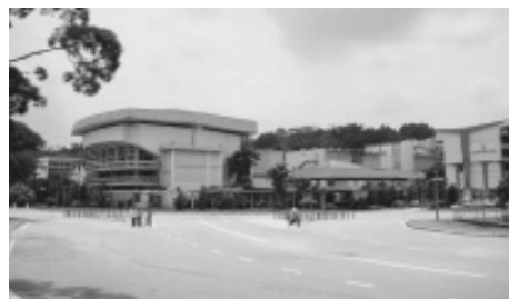
Figure 3: Main drop-off of Faculty of Science is facing the busiest junction in the campus.
