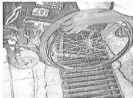
Figure 2: Gratings should be laid with the direction across the travel of wheels for the wheelchair users and can be avoided by short bridges (refer to Figure 6).
