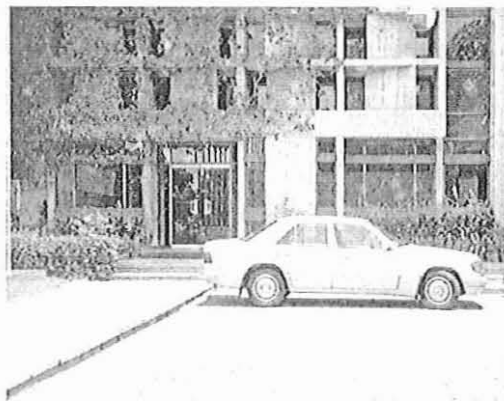
Figure 5a: Before construction of the ramp.
