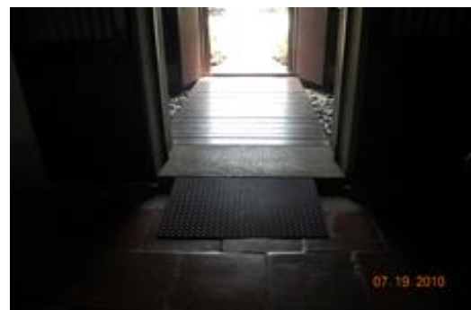
Fig. 5: Portable ramps at threshold of door way in Khoo Kongsi Museum
