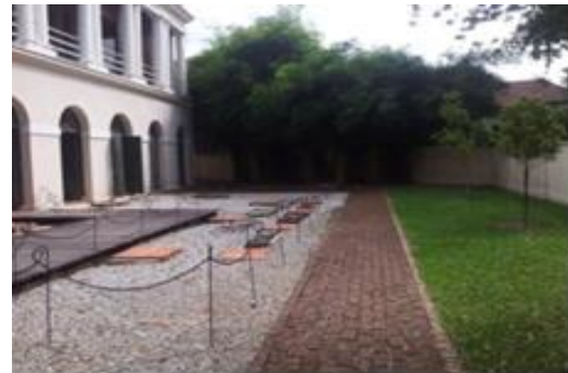
Fig. 3: Fair face brick pavement connects timber ramp to ancillary block at back yard
