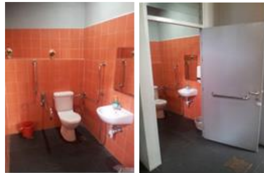
Fig. 9: Accessible toilet at the ancillary building block of Suffolk House
