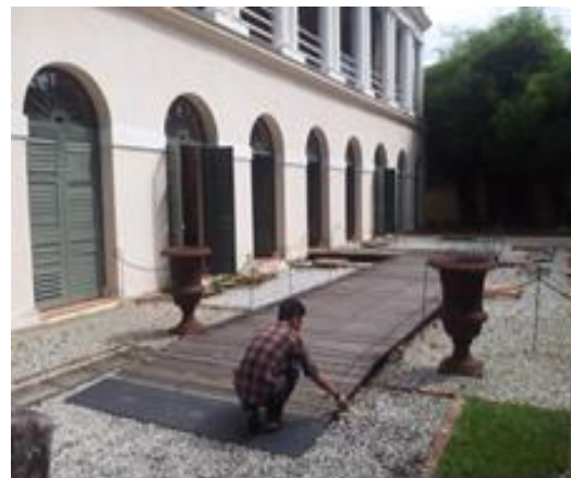
Fig. 7: Metal ramp to timber decking leading to main entrance of Suffolk House
