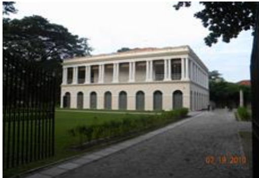
Fig. 2: Concrete pavement demarcates the accessible footpath
